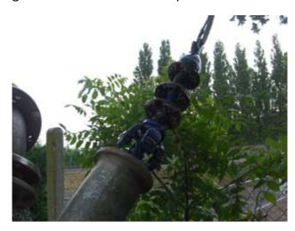
Pulling out a 6" mechanical cleaning tool
